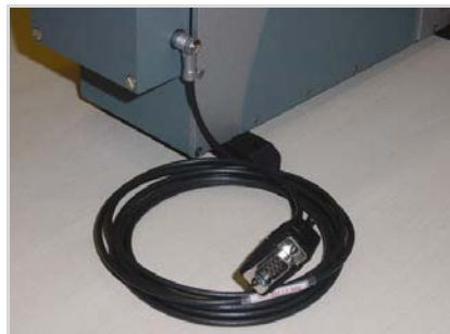
Figure 6: Shutter/Temperature cable connected to Mechelle
